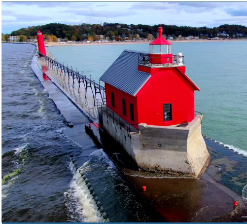
SOUTH PIERHEAD INNER LIGHTHOUSE
